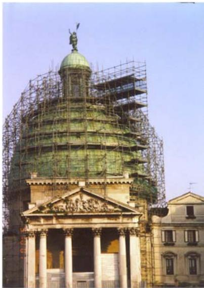
Fig. 0-2. The San Simeon Piccolo dome in Venice, Italy. The dome is surrounded with scaffolds, each of the metal rods has a diameter approximately 4 cm, 500 time smaller than the size of the dome, which has a diameter approximately 20 meters. Each of the rods serves as the construction scaffold for building or repairing the dome that is truly enclosed in 3-dimensions. The scaffold is eventually removed. Many proteins and other
