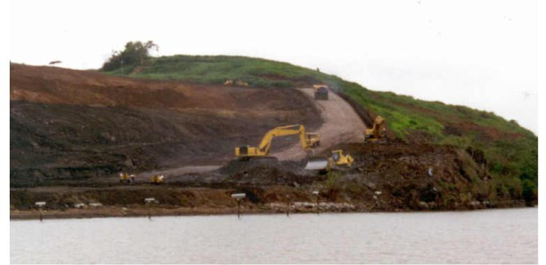
Widening the cut to allow large ships to pass safely
